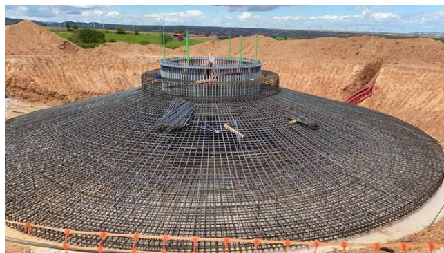
Figura 2.11 - Sapata circular [18]
