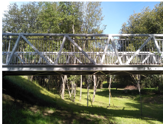
Figure 3.6: Picture of the pedestrian bridge in Parque da Asprela.
