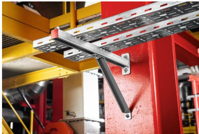
Fig.2.5 – Electrical application with Hilti's Typical structures.
