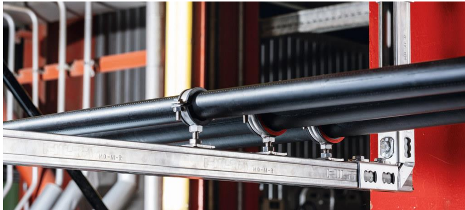
Fig.2.4 – Piping application with Hilti's Typical structures.
