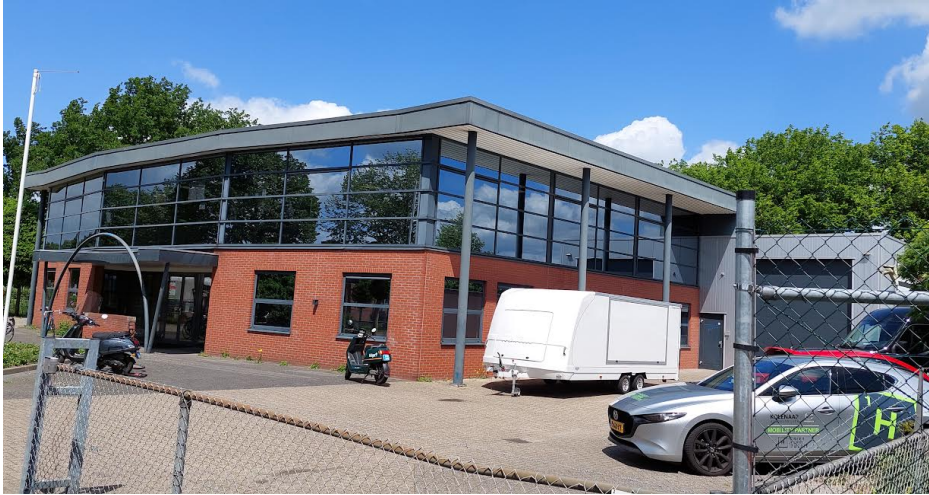
Figure C1 – Exterior view of the Future Factory.
