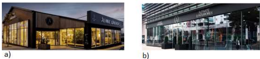
Fig. 2.3: Showrooms: a) Porto e b) Lisboa [2]
