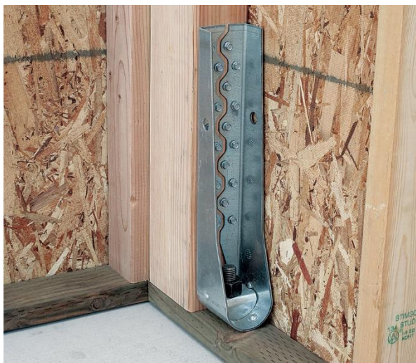
Figura 2.3. – Sistema “hold-down” (SIMPSON Strong-Tie)
