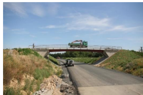
d) Friedberg Bridge over B3 Highway, híbrida de aço e GFRP [27]
