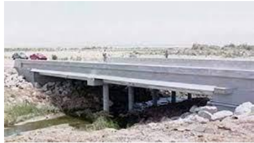
b) King's Stormwater Channel Bridge, GFRP [20]
