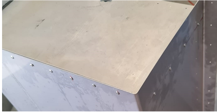
Figure 33: Rivet detail in the thermal chamber.
