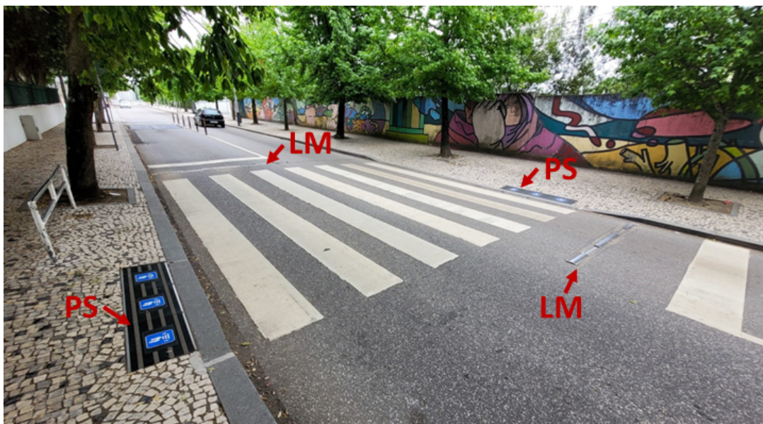
Figure 3.16: Pavnext pilot project in Matosinhos, Portugal
