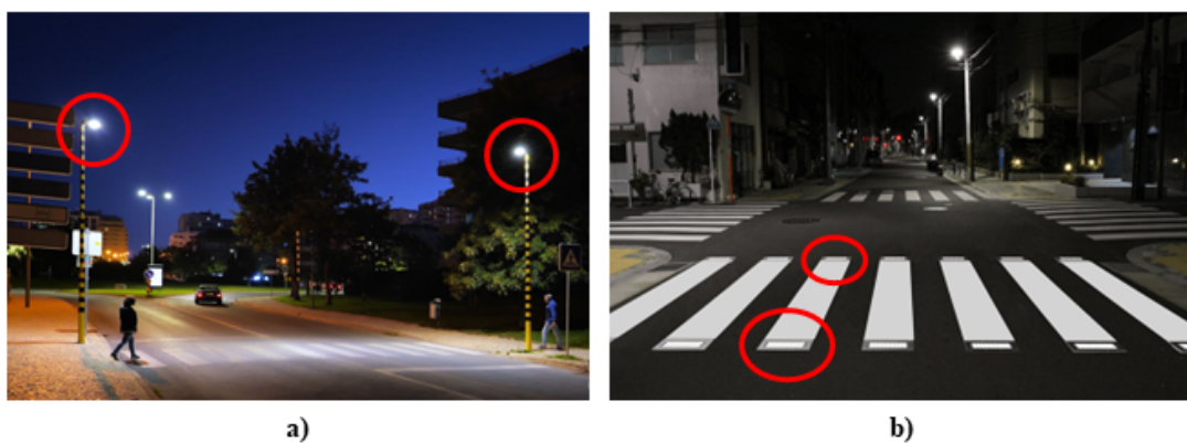
Figure 2.9: Constant light devices. a) NEOS LED; b) Sernis SR-CROSSLED-S. Adapted from: (Schreder, 2021), (Arminas, 2021)
