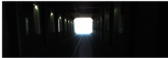
(b) Tunnel passage in sequence G. The low visibility degrades the performance of visual odometry techniques.
