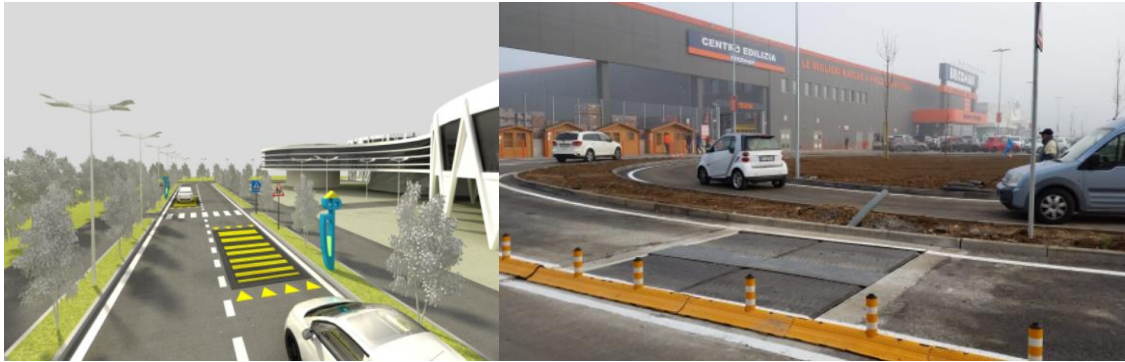
Fig.37- Lybra da Underground Power
