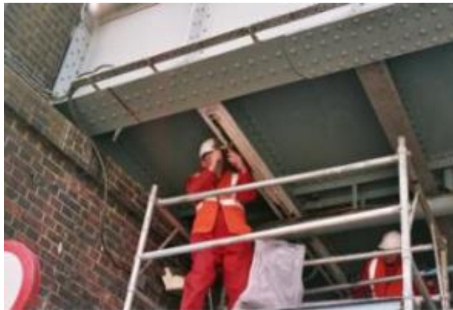
Figure 2-1: Application of CFRP to Acton Bridges, London (Harries, [1]).
