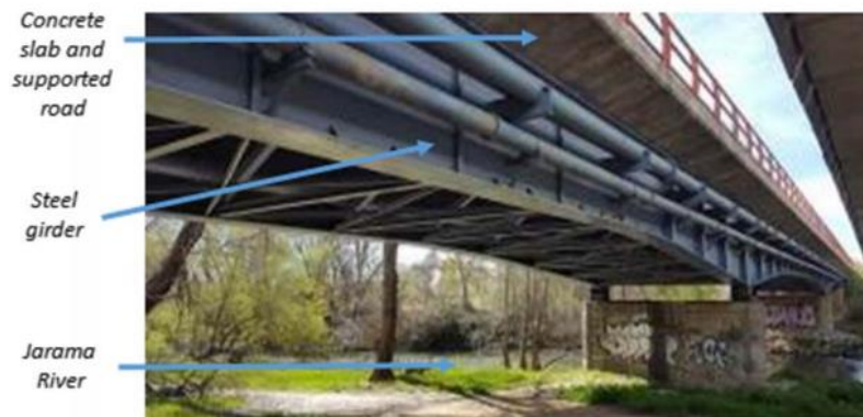
Figure 5-9: Jarama Bridge, Madrid.
