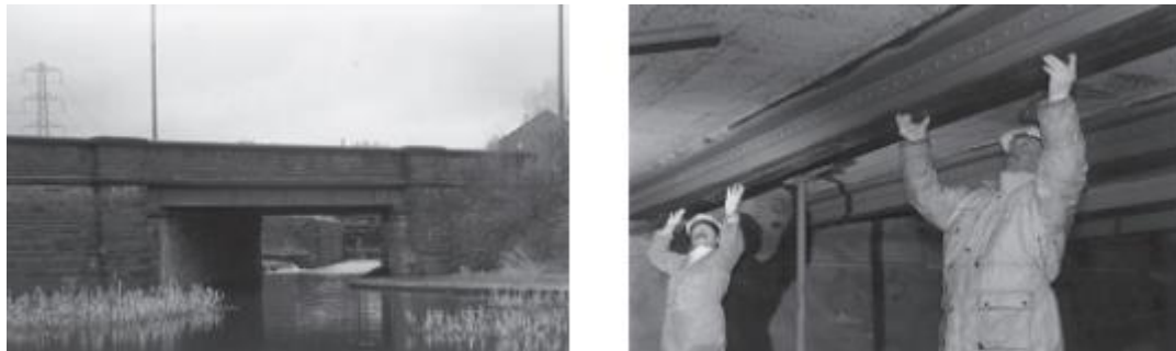
Figure 5-11: Slattocks Canal Bridge CFRP repair intervention.
