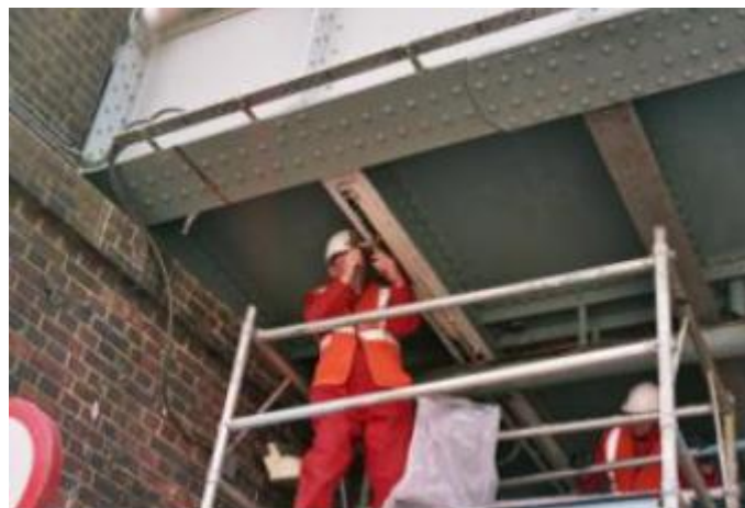
Figure 5-10: Fatigue strengthening of Acton Bridge using CFRP [32].
