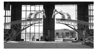
Fig. 1. 3D-printed steel bridge [1]
