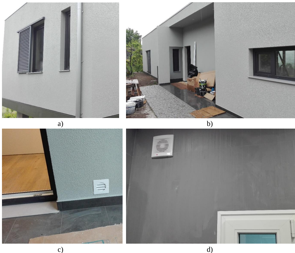
Figure 3.3. In-situ case study: a) and b) exterior openings; c) and d) examples of air extraction and admission points.
