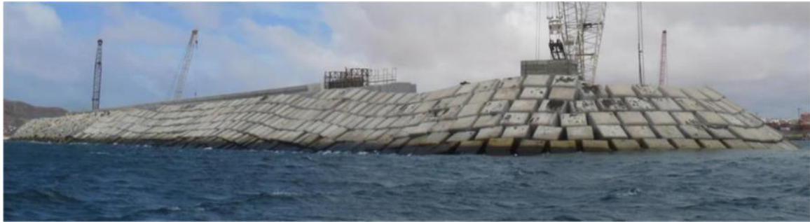
Figure 1.1 – Sal-Rei breakwater. Courtesy of Van Gent and van der Werf (2017).
