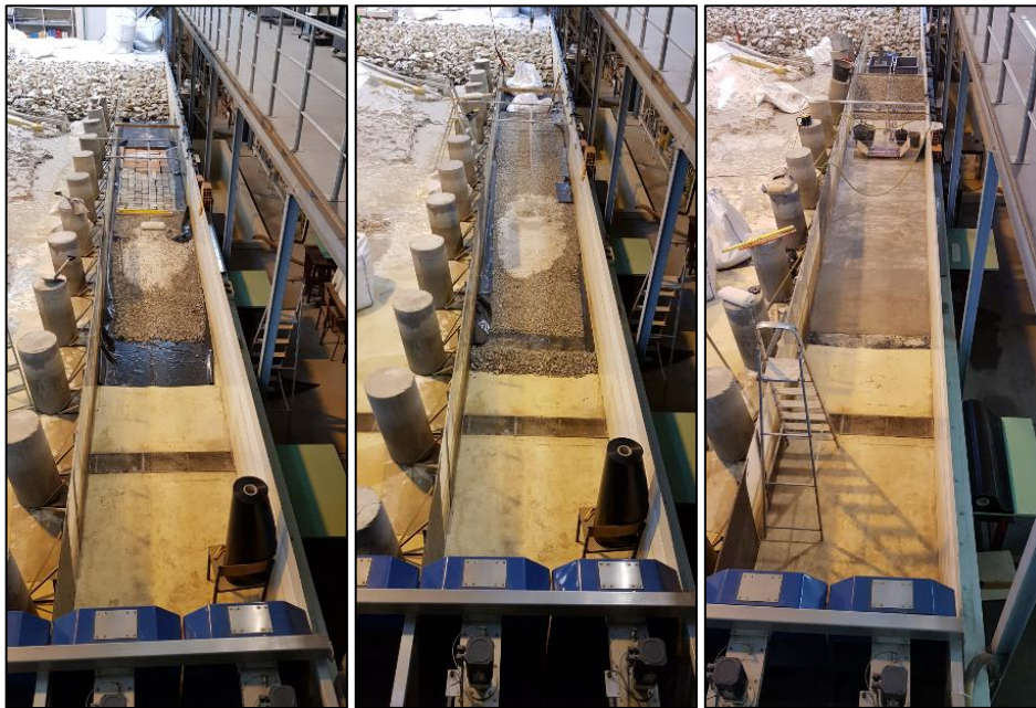
Figure 3.7 – Seabed construction sequence: Backfilling of the model area with bricks and blocks, and slope area with gravel (left); backfilling with gravel in the model area (middle); final step with concrete grout over backfilling (right).
