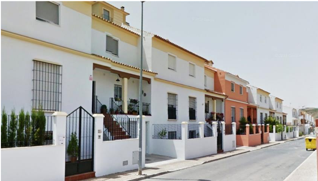
Figure 5.15 A view from the west part of the building fabric in the last phase of growth (1980 onwards) (Google Earth, 2020b)
