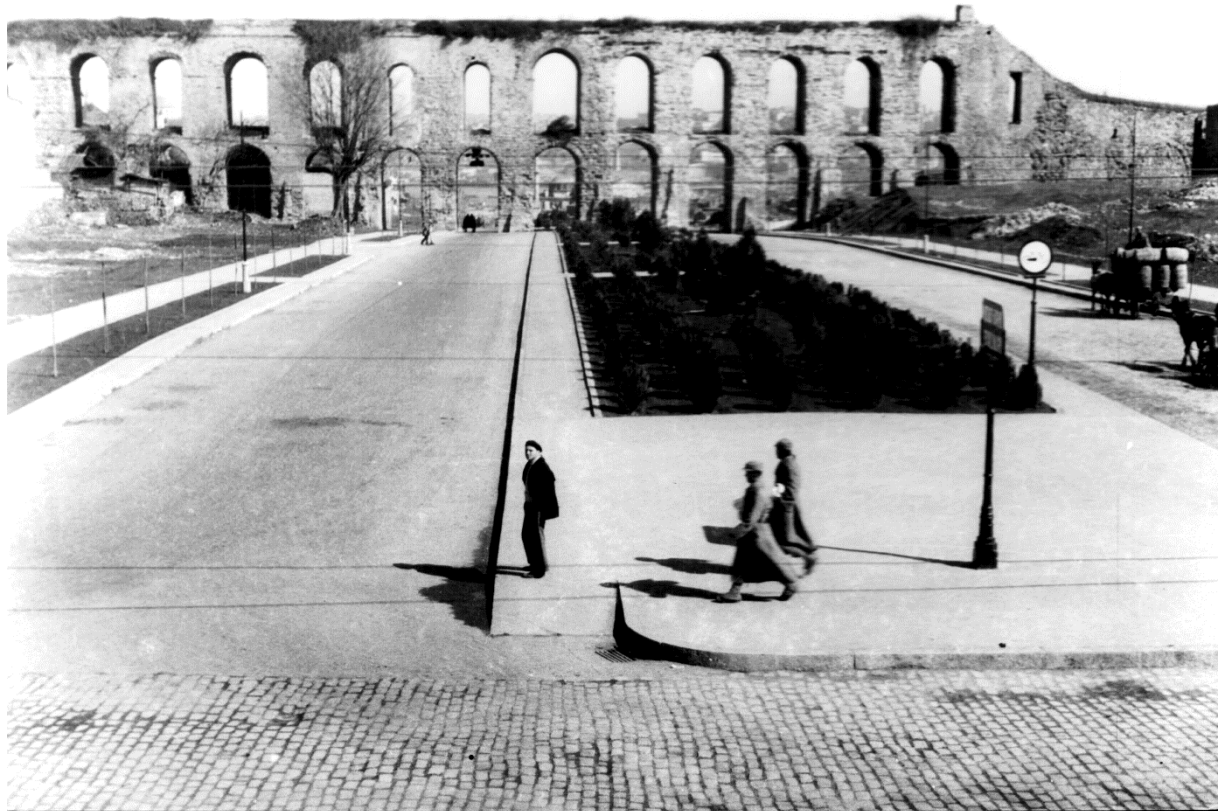
Figure 4.10 Valens Aqueduct in the 20 th century (IBB, 2019)
