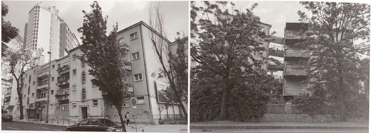
Fig. 12 and 13 Alvalade neighbourhood, Cells 1 and 2 (Lisbon, 1945–1948), Miguel Jacobetty Rosa–2066 dwellings, on the left. GPS: 38.752311N 9.146895W (left); Soda Póvoa neighbourhood (Vila Franca de Xira, 1953), Nuno Teotónio Pereira–12 dwellings. GPS: 38.859693N 9.067165W (right). Photos by Gisela Lameira (2018).
