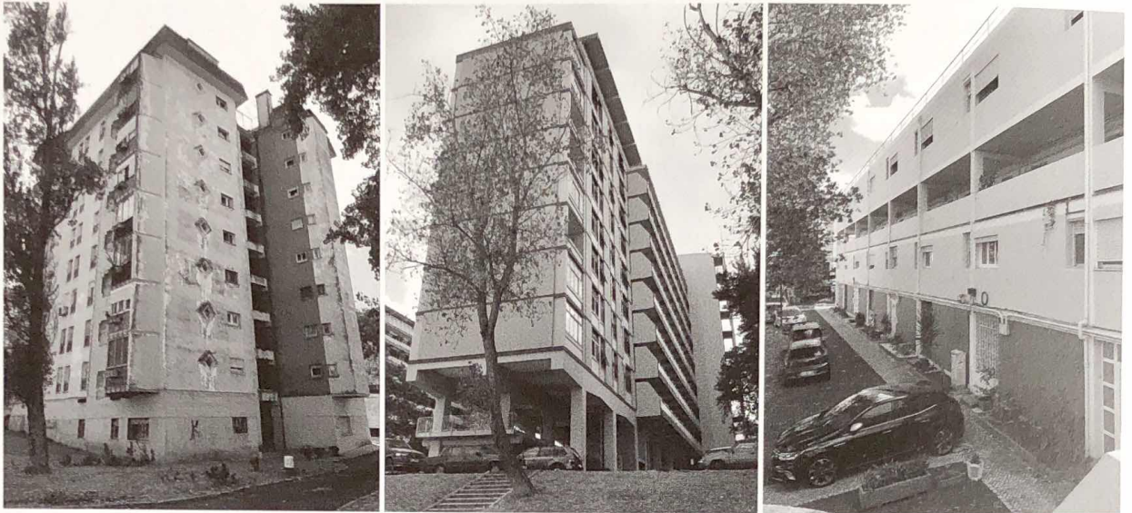
Fig. 23, 24 and 25 Cell A-Cat. II (Lisbon, 1957–1968), Nuno Teotónio Pereira, Nuno Portas, António Pinto de Freitas–384 dwellings. GPS: 38.776181N 9.116921W (left); Cell A-Cat. III (Lisbon, 1959–1964), Cândido Palma de Melo, Artur Pires Martins–128 dwellings. GPS: 38.775414N 9.114904W (middle); Building type IID (Lisbon, 1958–1960), Pedro Cid, Fernando Torres et al.–80 dwellings. GPS: 38.776376N 9.114732W (right). Photos by Gisela Lameira (2018).
