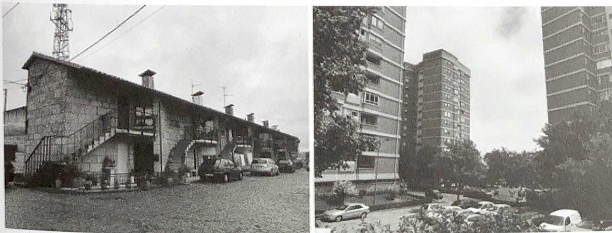
Fig. 10 and 11 Santa Marta neighbourhood (Barcelos, 1955–1962), Nuno Teotónio Pereira—20 dwellings. GPS: 41.534584N 8.608408W (left); Torres vermelhas da Pasteleira (Porto, 1966–1972), João Serôdio, Luís Almeida d'Eça, Rui Paixão—500 dwellings, on the right. GPS: 41.1513384N 8.6630958W (right) Photos by Gisela Lameira (2018).
