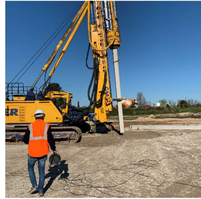
Figure 4: Impact pile driving at the experimental test site.
