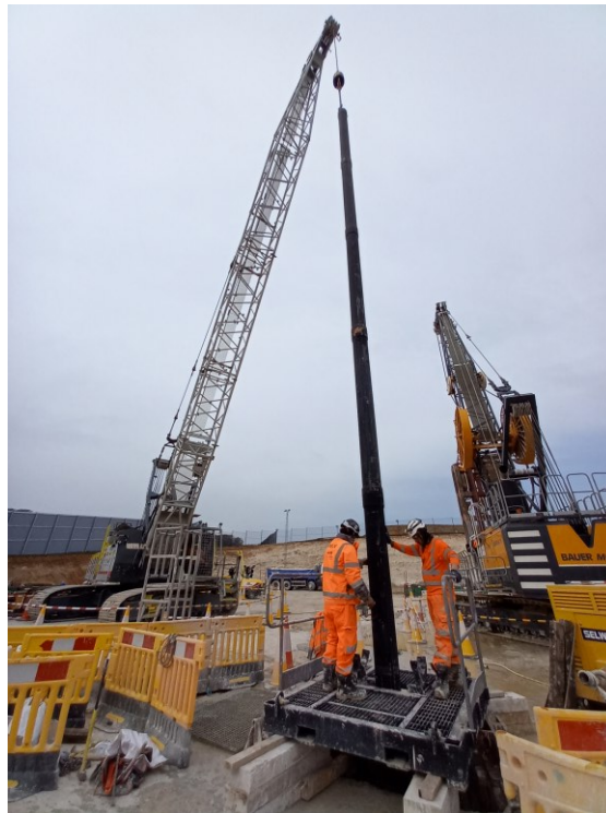
Figure 23: Tremie pipes installation
