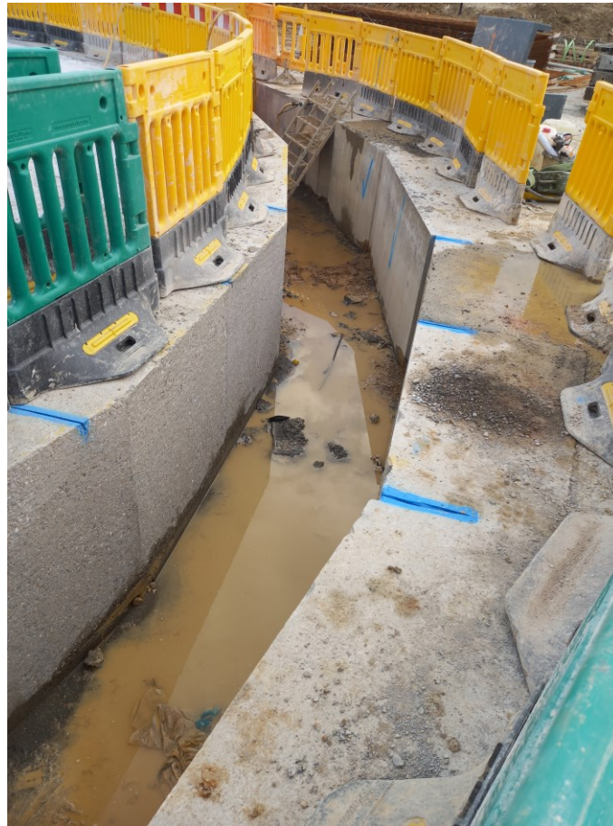
Figure 9: Guide wall before backfilling
