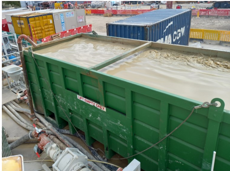
Figure 26: Freshly mixed bentonite in mixing tank
