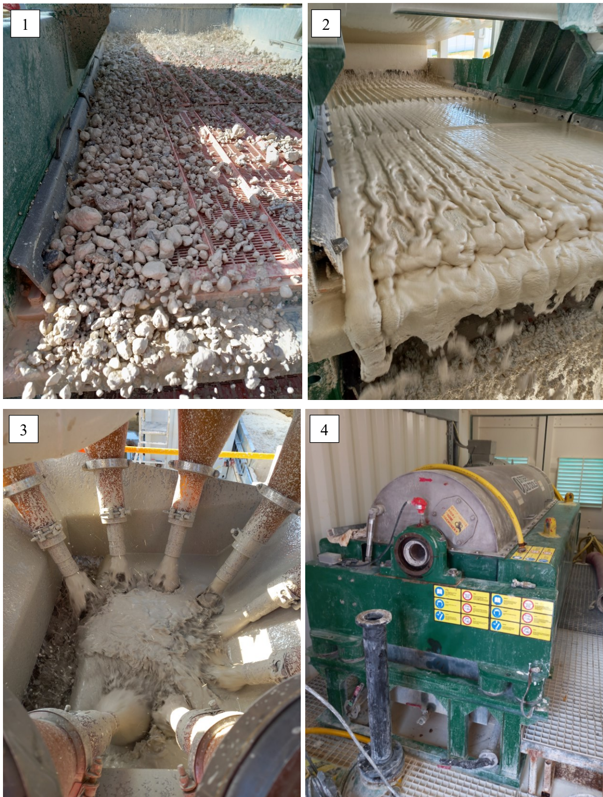
Figure 37: Recycling set up component: 1-Vibrating screens (first set); 2-Vibrating screens (second set); 3- Hydrocyclones; 4- SOBB55 Centrifuge
