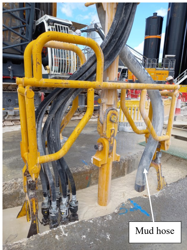
Figure 27: Cutter partially submersed in bentonite fluid during panel excavation
