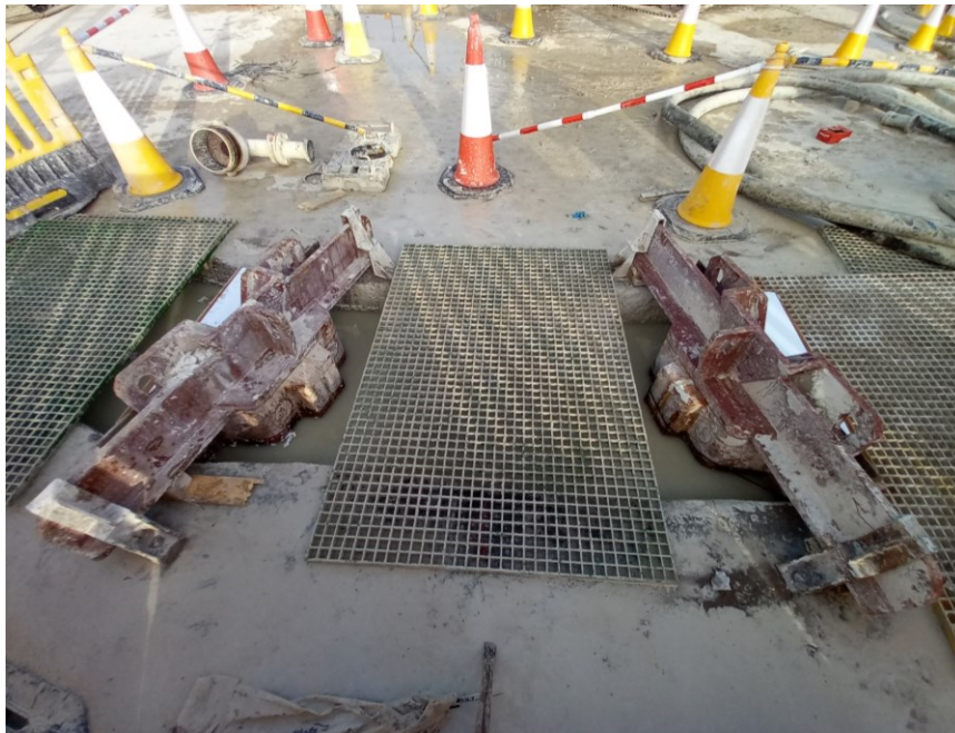
Figure 13: Concreted panel with stop ends installed
