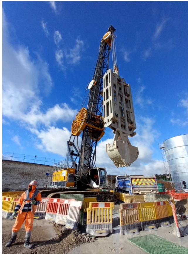
Figure 16: Hydraulic Grab bucket full of material ready for evacuation
