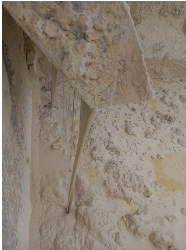
Figure 39: Centrifuge decanting solid waste discharging point during excavation
