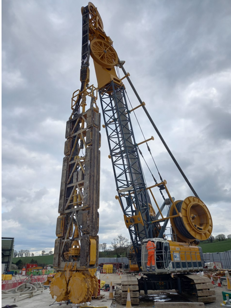
Figure 18: Cutter ready after assembly
