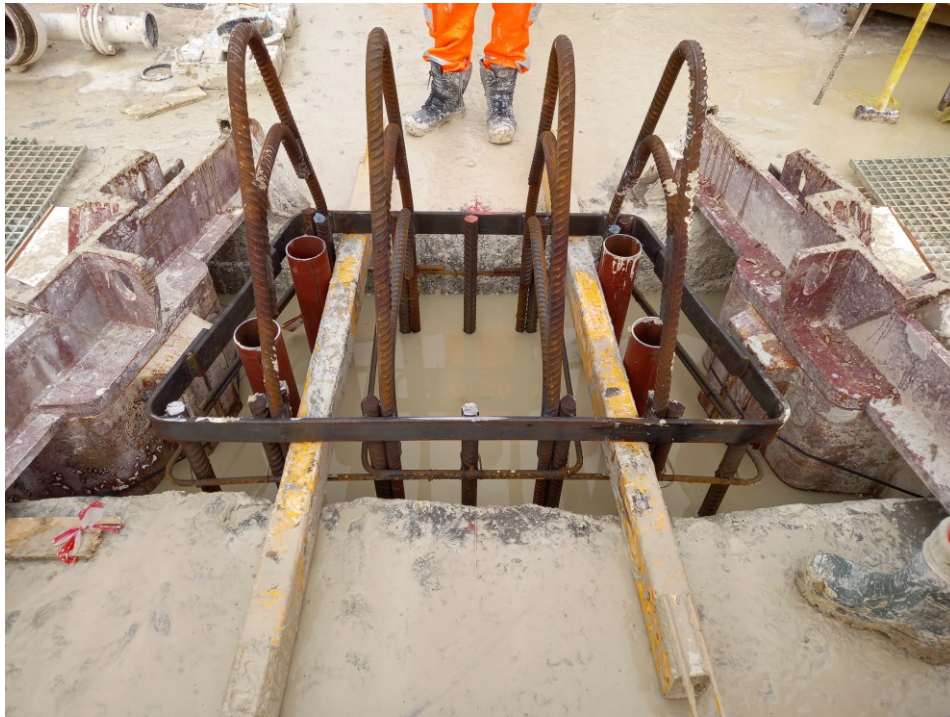
Figure 21: D-wall reinforcement cage installation (1 bite primary panel, stop ends on the sides)
