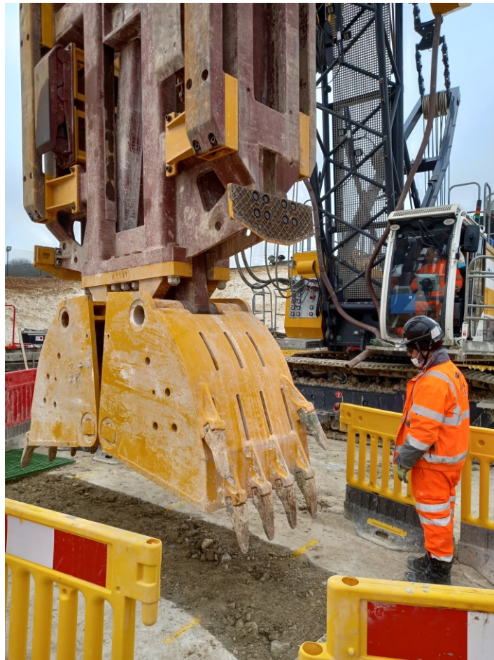
Figure 15: Start of hydraulic Grab excavation
