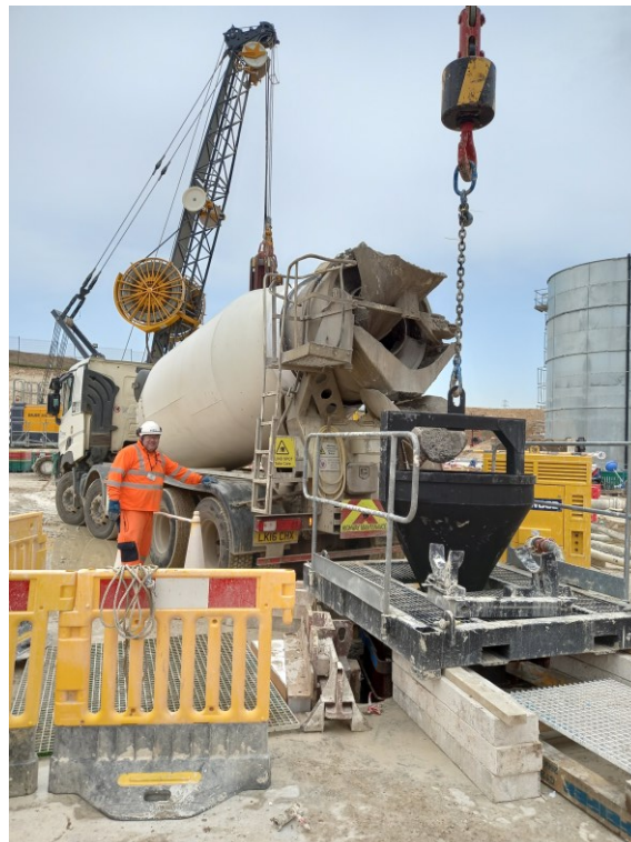
Figure 24: Panel concrete pouring
