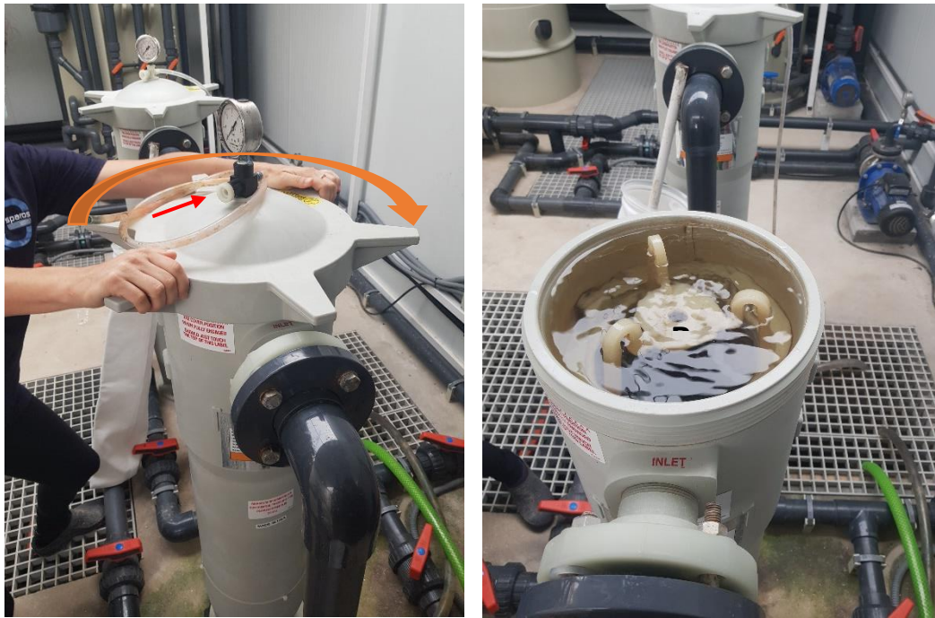
Figure 2 - Mechanic filter opening (arrow - pressure valve / big arrow - opening movement) B – Filter holder.
