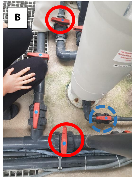
Figure 1 – A – Mechanical filter valves opened (circle – inlet and outlet valves / stripped circle – sewer valve closed opened) / B – Mechanical filter valves(closed) and sewer valve (opened) during the procedure.
