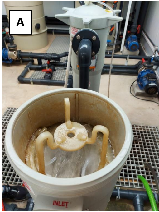
Figure 4. A- Filling the mechanic filter, B - final valves position.
