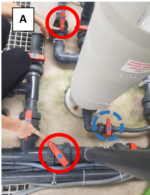
Figure 1 – A – Mechanical filter valves opened (circle – inlet and outlet valves / stripped circle – sewer valve closed opened) / B – Mechanical filter valves(closed) and sewer valve (opened) during the procedure.
