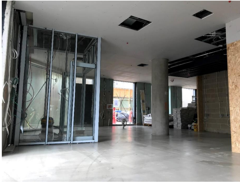
Fig. 4.2 - Common area on the ground floor of the building, coffee shop. Still under construction at the date of this publication – Source: Regal Homes London
