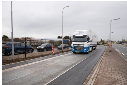
Figure 2.4: SolaRoad's photovoltaic pavement surface in Haarlemmermeer (NL), 2019 (extracted from SolaRoad 2 )
