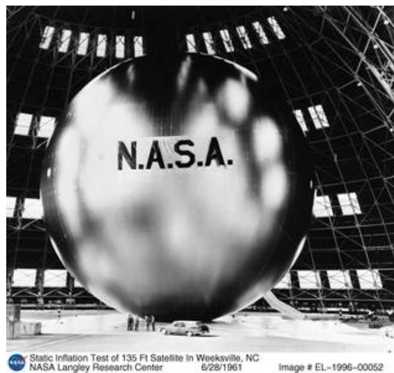
Figure 2.1: Echo 1 ground inflation test, credits: NASA
