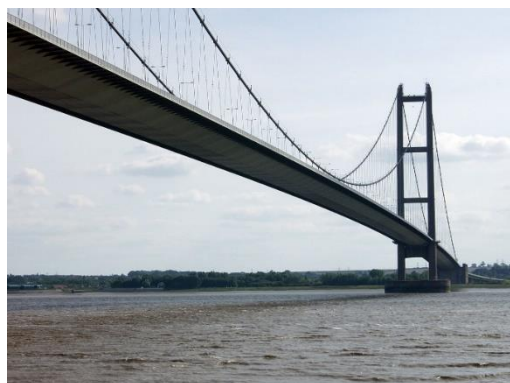
Figura 25 - Humber Bridge (1981), Lincolnshire, Reino Unido (vão livre de 1410m)
