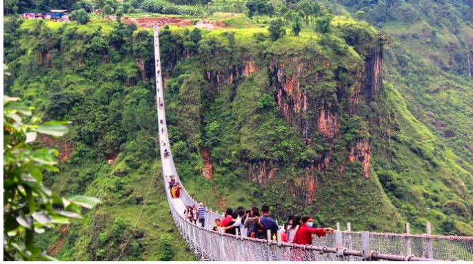
Figura 28 - Baglung Pargat Footbridge (2020), Nepal (vão livre de 567m)
