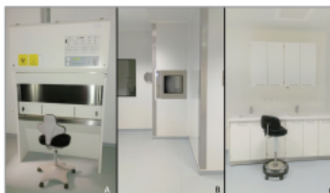
Figure 2. Girassol Clinic oncology pharmacy unit. (A) Primary engineering control (BSC type II) in buffer room. (B) Pass through with HEPA filters. (C) Anteroom (making ready area) meeting USP 797 criteria.
