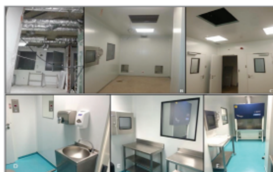
Figure 3. Sagrada Esperança Clinic oncology pharmacy unit before and after construction. Before: (A) Building (making of) HVAC to the buffer room. (B) Building the buffer room in modular construction. (C) Building the anteroom in modular construction. After construction meeting USP 797 criteria [36]: (D) Final anteroom. (E) Final anteroom (making ready area) connected through a pass through to the buffer room. (F) Final Buffer room with BSC type II B2.
