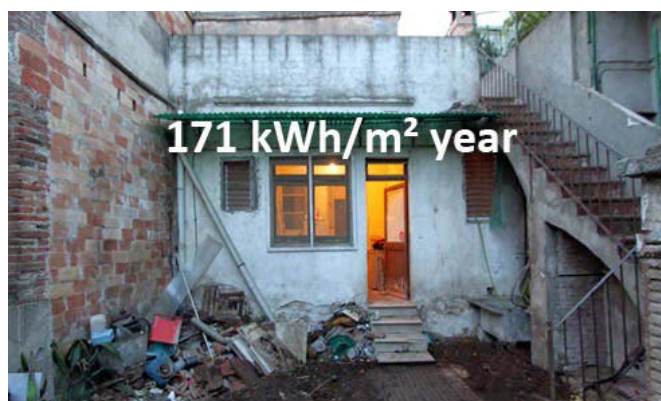
#70 . Low Energy MZ House. Aatoria: Calderon Folch Studio.
