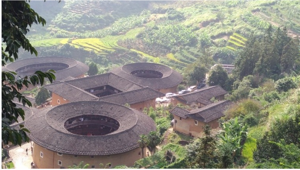
Figure 2. View of a Tulou cluster.
