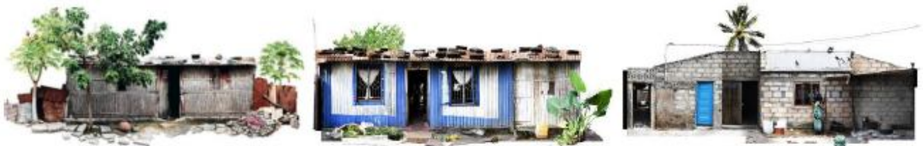
Figure 11. The three constructive forms in Maputo's SPN: the reed house (left); the zinc plate house (middle); the cement block house (right). Source: Eskemose and Mottelson (2016: 13).
