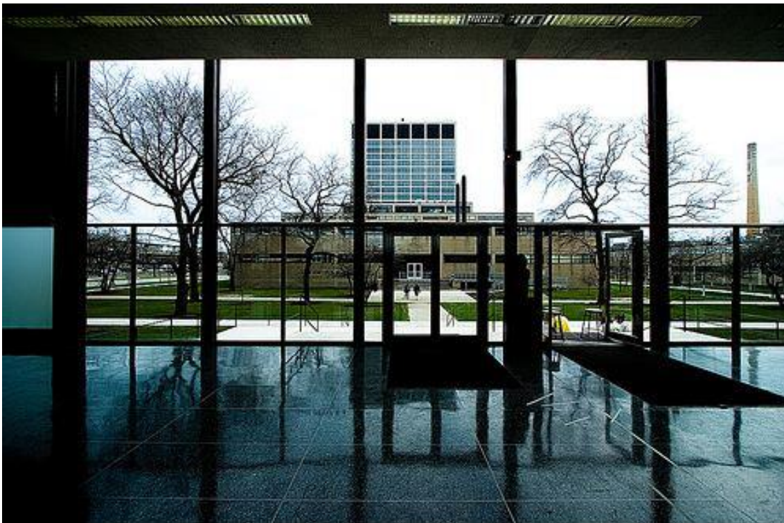
[A88] Mies van der Rohe 1950 – 1956, IIT, Crown Hall , Illinois Institute of Technology.
