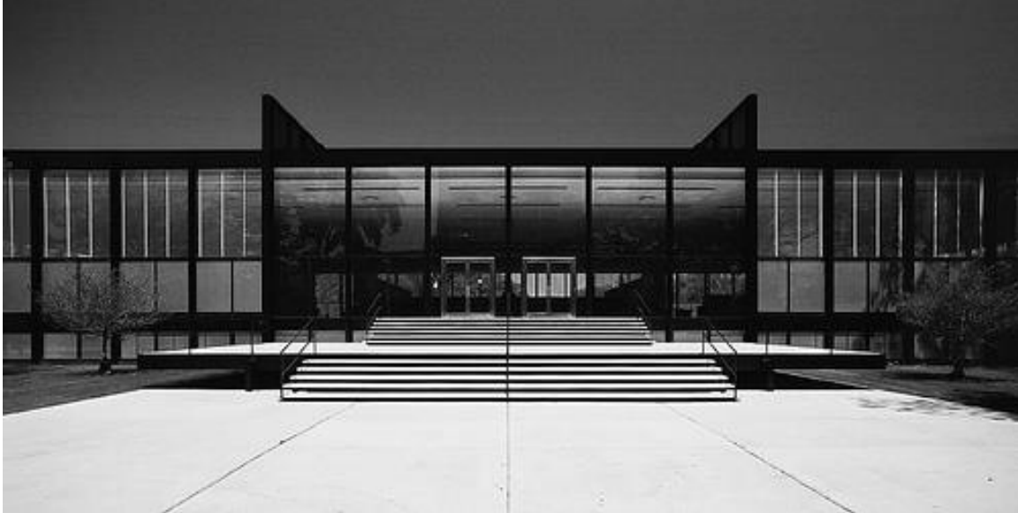
[A87] Mies van der Rohe 1950 – 1956, IIT, Crown Hall , Illinois Institute of Technology.
