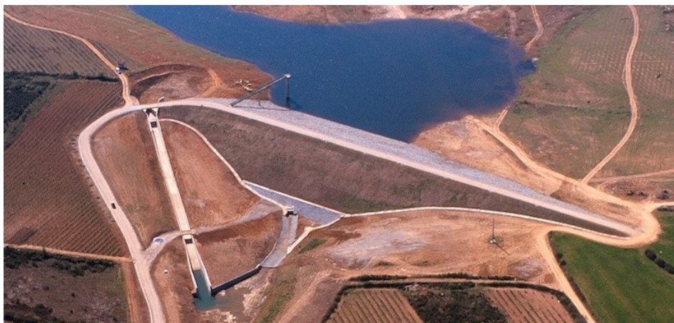
Fig. 6 - Chute spillway of the Vermiosa dam on the right hillside, Guarda, Portugal, 1999 (web 3 Nov 2016 www.mota-engil.pt ).
