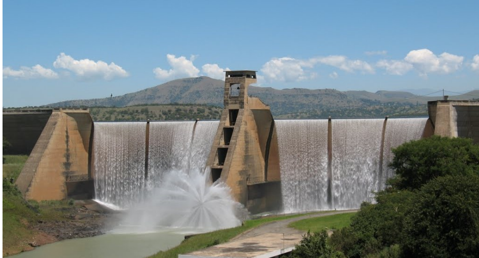
Fig. 4 - Downstream view of the 40m-high Wagendrift dam, Estcourt, South Africa, 1963 (photo credit: Neil Overy).
