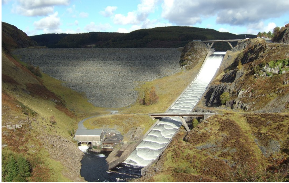
Fig. 14 - Roll waves in the spillway of the Llyn Brianne Rock-fill Dam, Wales, United Kingdom (copyright © Geoffrey Davies).
