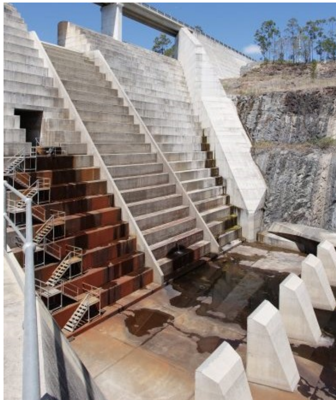
Fig. 9 – Stepped spillway of the Hinze dam, South East Queensland, Australia 1976, (copyright ©Hubert Chanson 2014).
