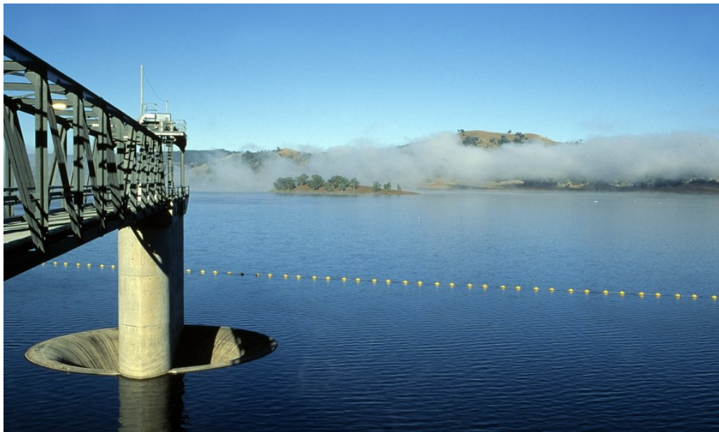
Fig. 7 - Shaft spillway intake of the Chaffey dam, located at New South Wales, Australia, 1979, (photo credit: Brad Sherman).
