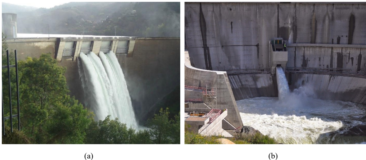
Fig. 105 – (a) Caniçada dam impinging jets (Image from www.meteopt.com , forum ( https://www.meteopt.com/forum/topico/seguimento-rios-e-albufeiras-2014.7457/pagina-2 )). (b) Bottom outlet jet of the Baixo Sabor dam, Portugal, 2016 (image from https://akisabor.blogspot.com/2014/04/descarga-de-fundo.html )
