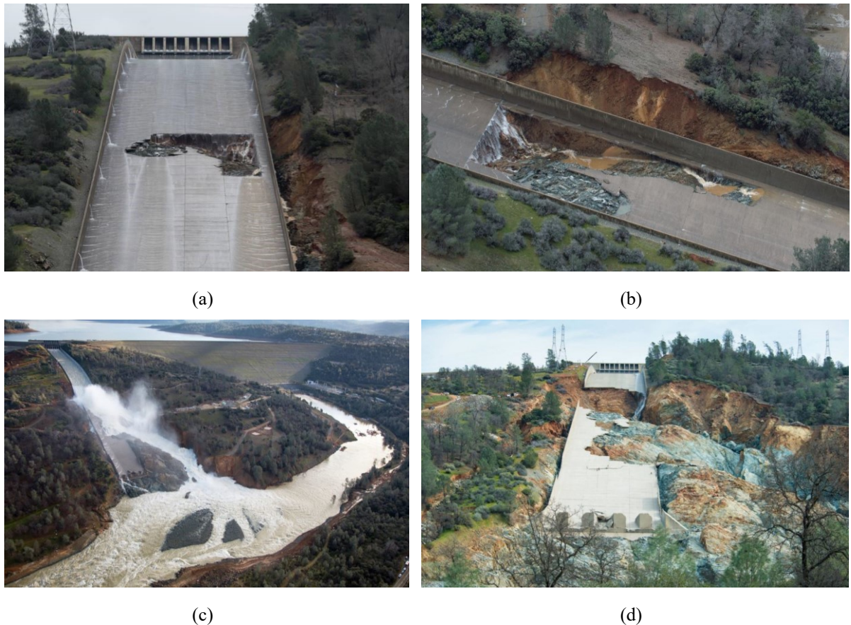
Fig. 17 – Evolution of the Oroville spillway failure in chronological order from (a) to (d). Photographs from Williamson (2017).
