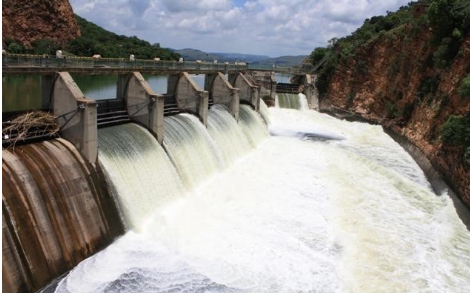
Fig. 11 - Free-surface aeration in the spillway of Hartbeespoort Dam, North West Province, South Africa, 1923 (web 3 Nov 2016 www.ewiza.co.za ).
