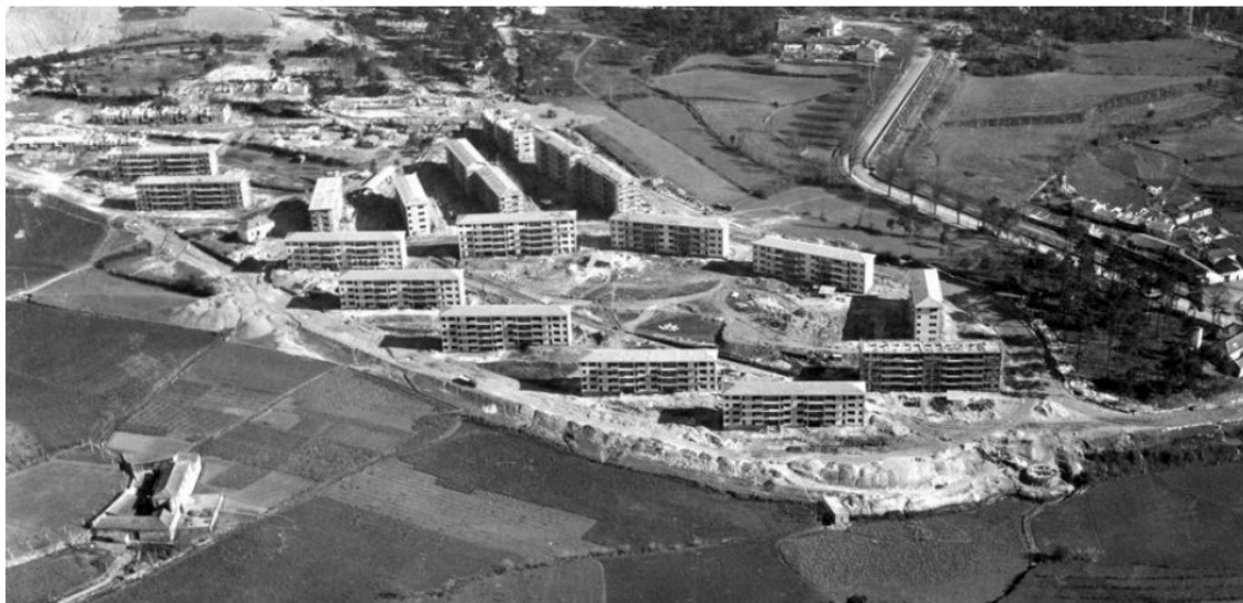
Fig. 2. Cerco housing complex. Construction phase, 1961 (Arquivo Histórico Municipal do Porto)
