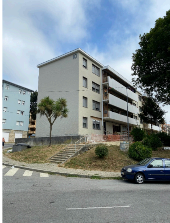
Fig. 11. Intervention by José Gigante. Block 10 (under construction). (Luciana Rocha, 2020)
