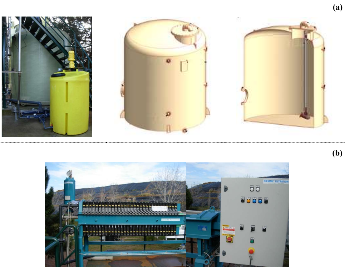
Figure 4.11 – Photograph and 3D schematic images of (a) sludge tank and (b) filter-press system.
