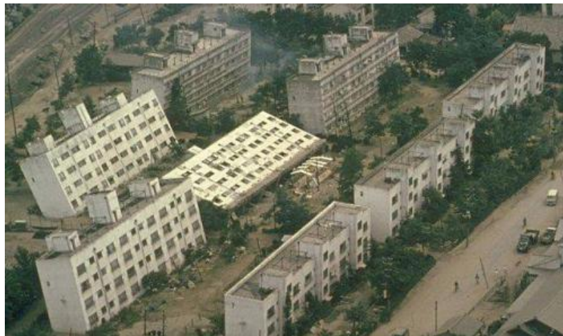
Figure 2.5. Niigata Earthquake, 1964 (Ungtss, 1964).
