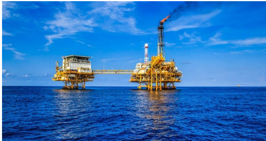
Figure 2.3 Onshore wind farms(a); Offshore oil and gas facilities, (b).
