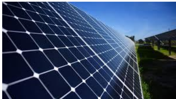
Figure 3.25 - PV solar panel composed of several PV cells
