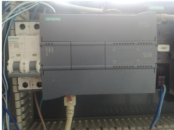
Figura 5.9 - PLC s7-1200 com a CPU1215C DC/DC/DC.
