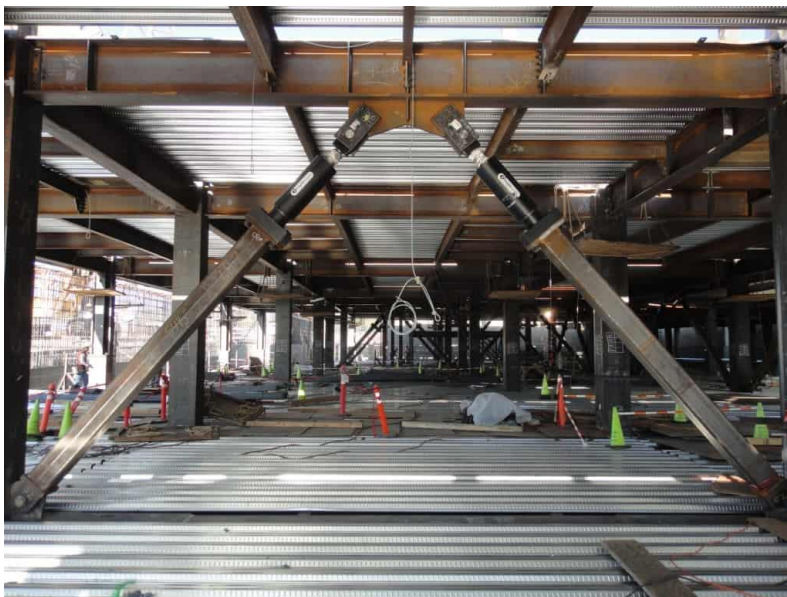
Figure 2 - Application of fluid viscous dampers on buildings: San Bernardino Justice Center (SBJC) – California, USA [13].
