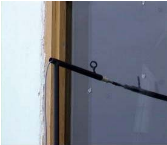
Figure 3-16: A view of the new method for the anemometer insertion
