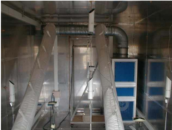
Figure 6-26: "building" model (photo)
