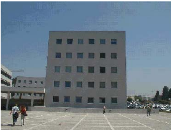
Figure 7-4: South Façade of the building
