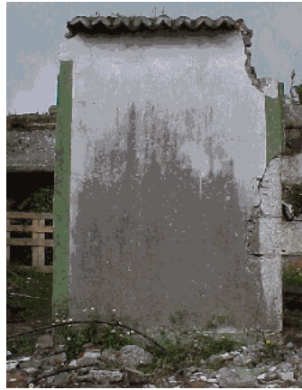
Fig. 4.3 – Parede original (A1)
