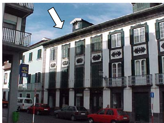
a) Fachada principal
