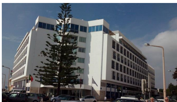
(a) Fachada principal
