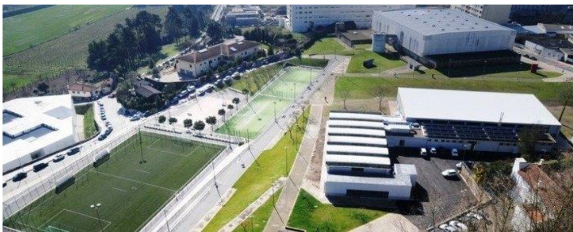
Figura 8 – Complexo Desportivo Municipal ( https://www.cm-stirso.pt/viver/desporto/complexo-desportivo-municipal ).
