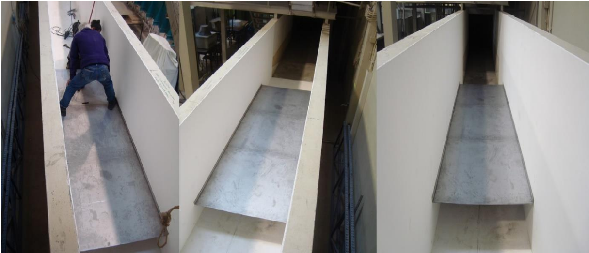
Figure 3.9 - Stage 4: Installation of the metallic plate.
