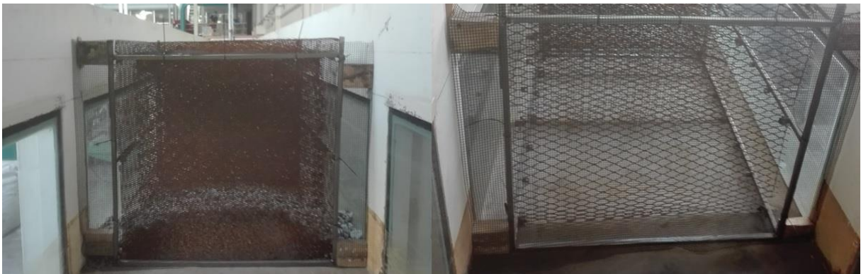
Figure 3.45 - Plastic net at the downstream and upstream box faces.
