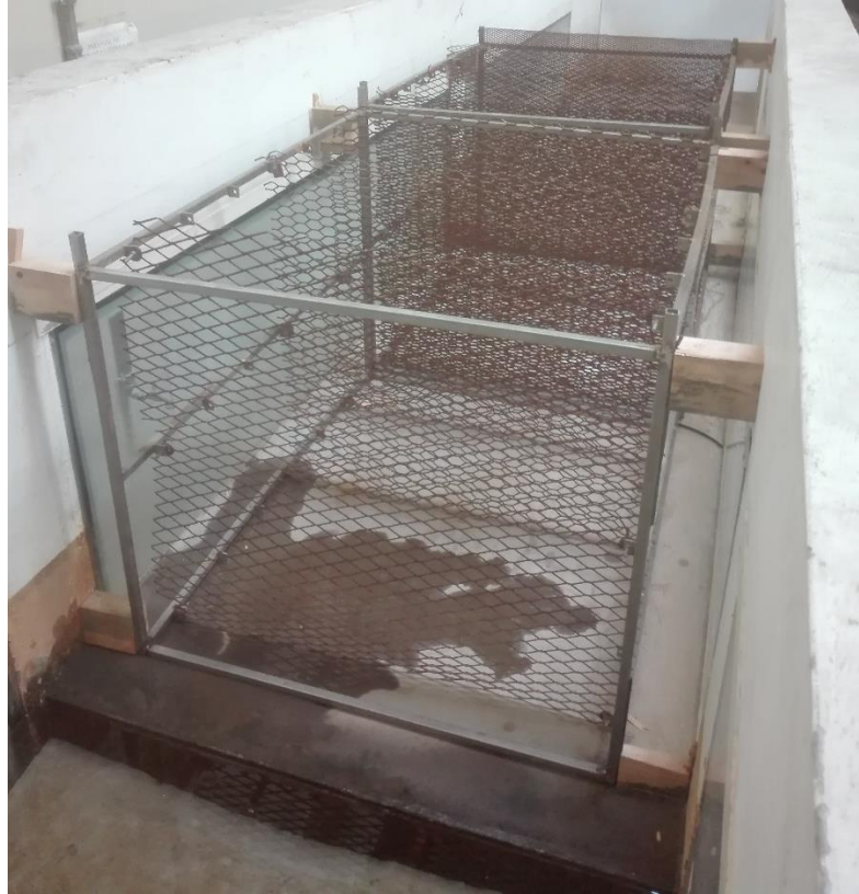
Figure 3.44 – Boxes fixing to the flume walls.
