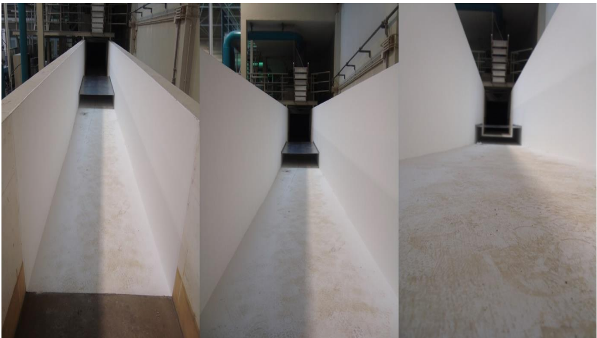
Figure 3.10 – Flume reconstruction stage 4 conclusion.
