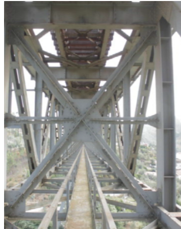
Figure 4.2: Photo of the interior of the 3D truss of the deck (Infraestruturas, 2018).
