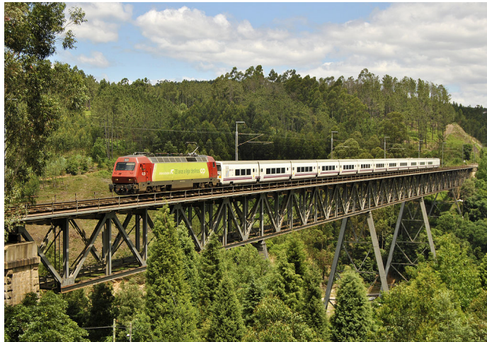
Figure 4.1: West view of Várzeas railway bridge (Infraestruturas, 2018).
