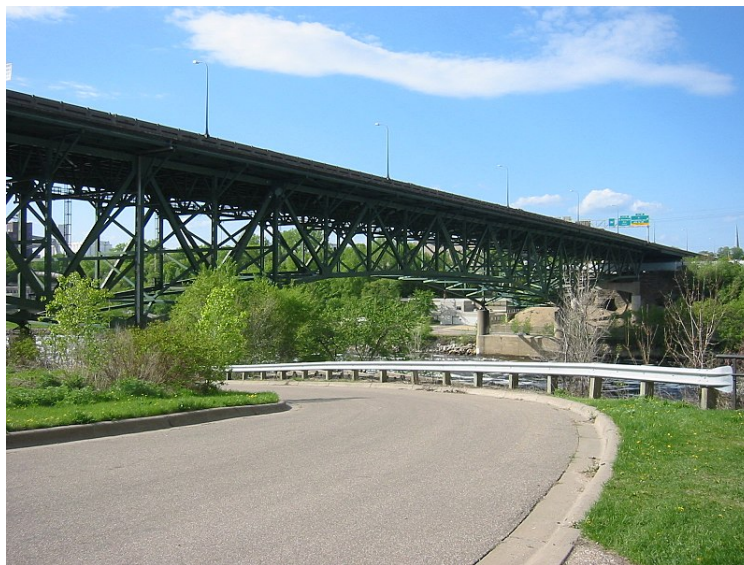
Figure 2.14: Bridge I-35W, Minneapolis, Minnesota, USA, 2006 (photographed by I. Elkman).
