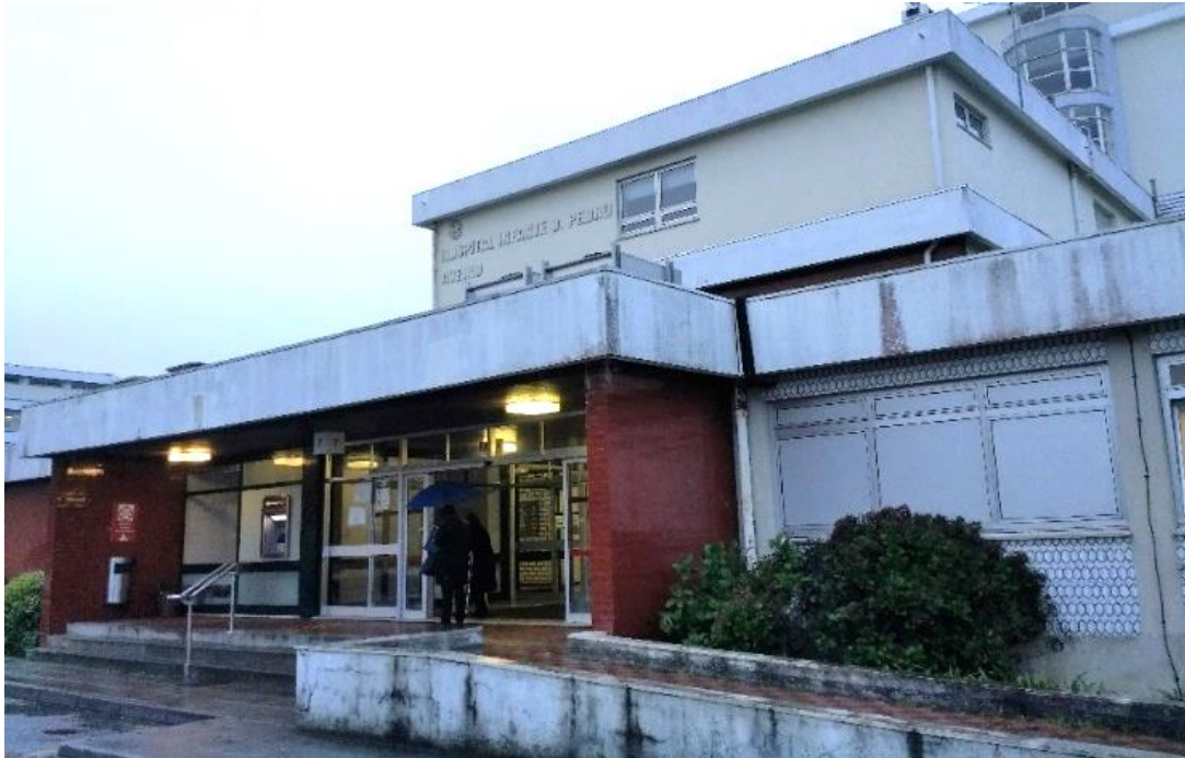
Figure 80 - Main entrance of hospital C - Infante D. Pedro, in Aveiro
