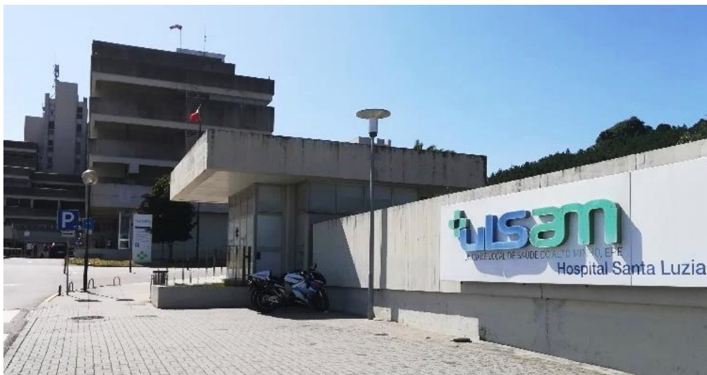
Figure 78 - Entrance of hospital A - Santa Luzia, Viana do Castelo
