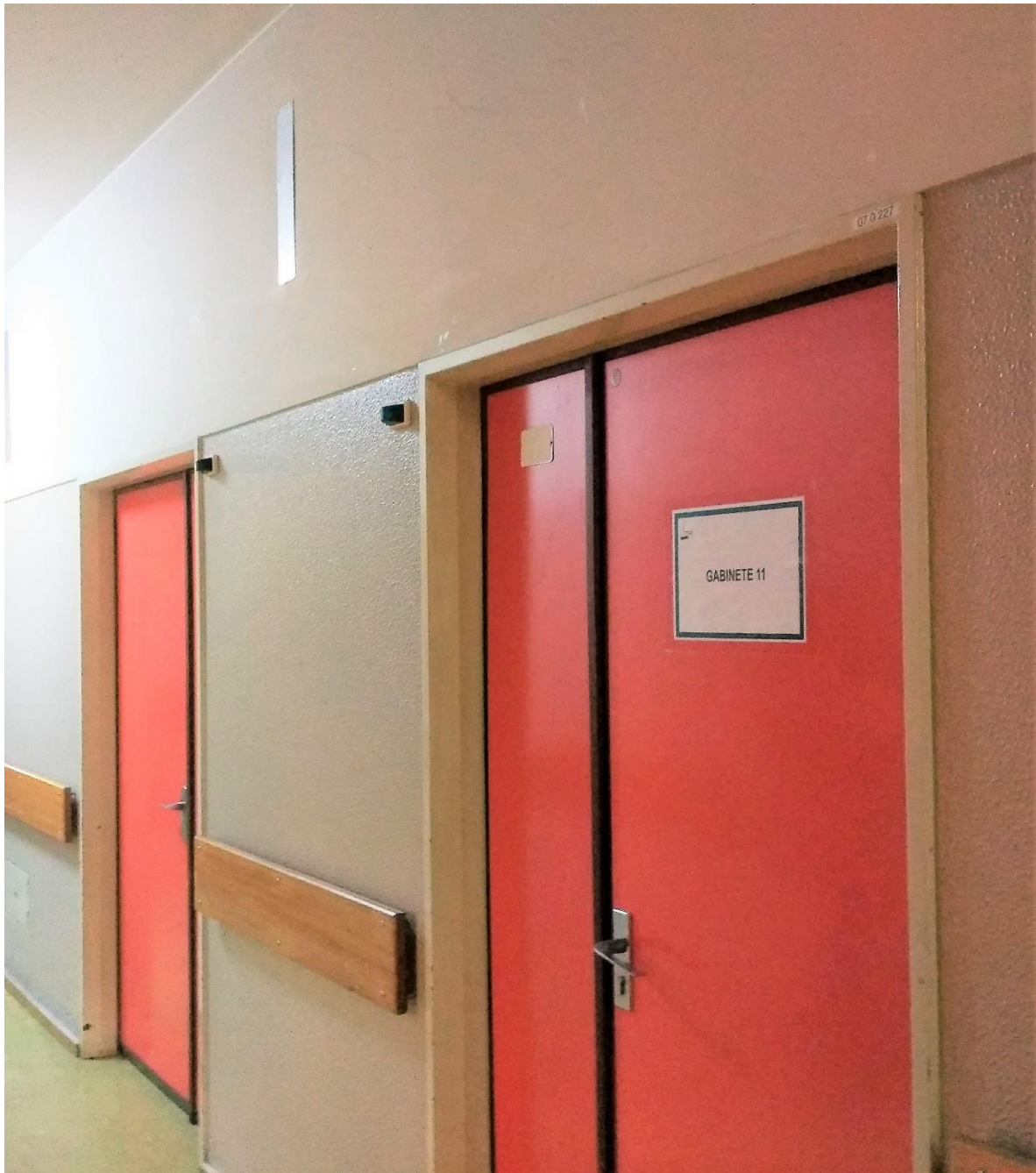
Figure B6 - Identification/Locational signage indicating the doors of the medical offices at hospital C
