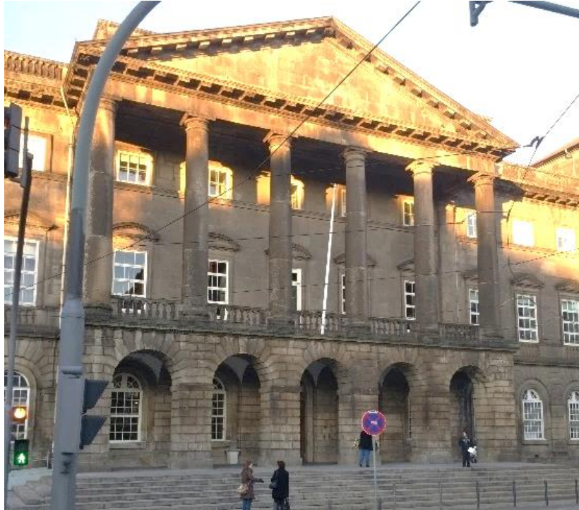
Figure 79 - Main entrance of hospital B - Santo António, in Porto
