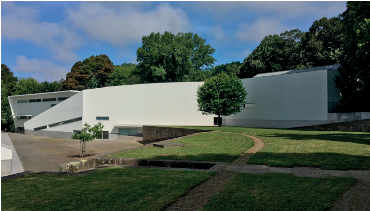
Figure 3. Álvaro Siza, Faculty of Architecture, Porto, Portugal, conservation 2016-2017. © Simone Ruivo, 2017.
