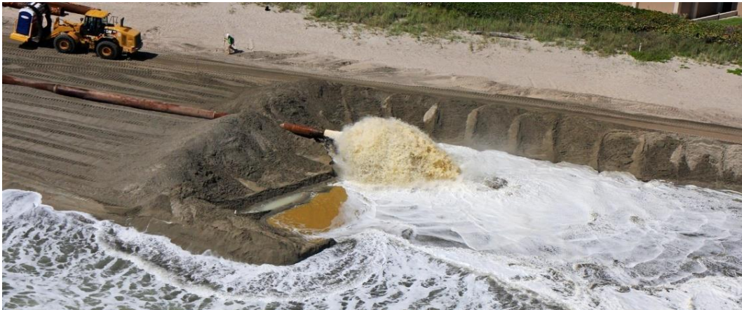
Fig. 2.5 - Beach nourishment (Martin County Florida).
