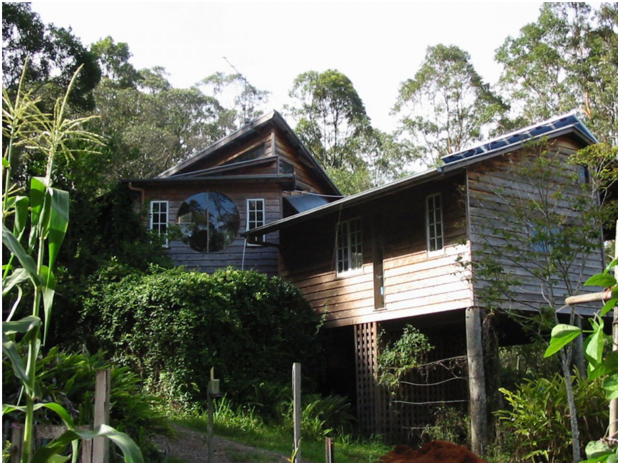
Fig.45 - Solar House, Crystal Waters
