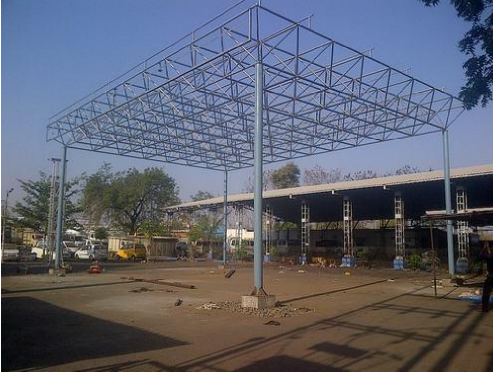
Figure 16 Example of Spaceframe construction (temporary accomodation) (11)
