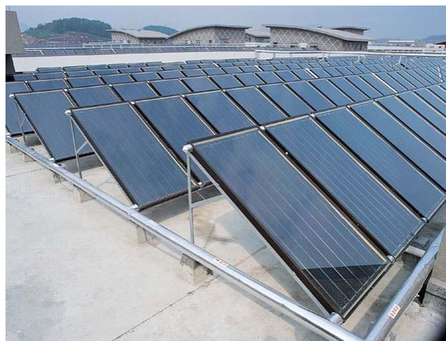
Figure 14 - Flat plate solar collectors mounted in a flat roof. Extracted from [37].
