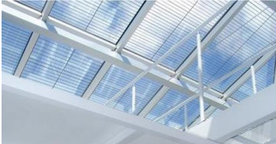
Figure 11 - Window-integrated PV. Extracted from [42].
