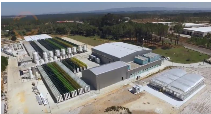
Figure 1. 1. Industrial facilities of Algafarm.
