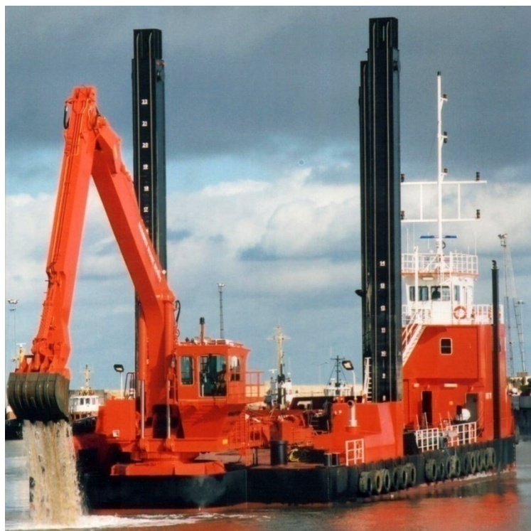
Figure 8 | Backhoe during dredging works
