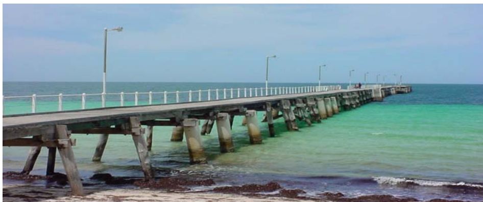
Figure 4 | Existing structures can provide support for bypassing equipment
