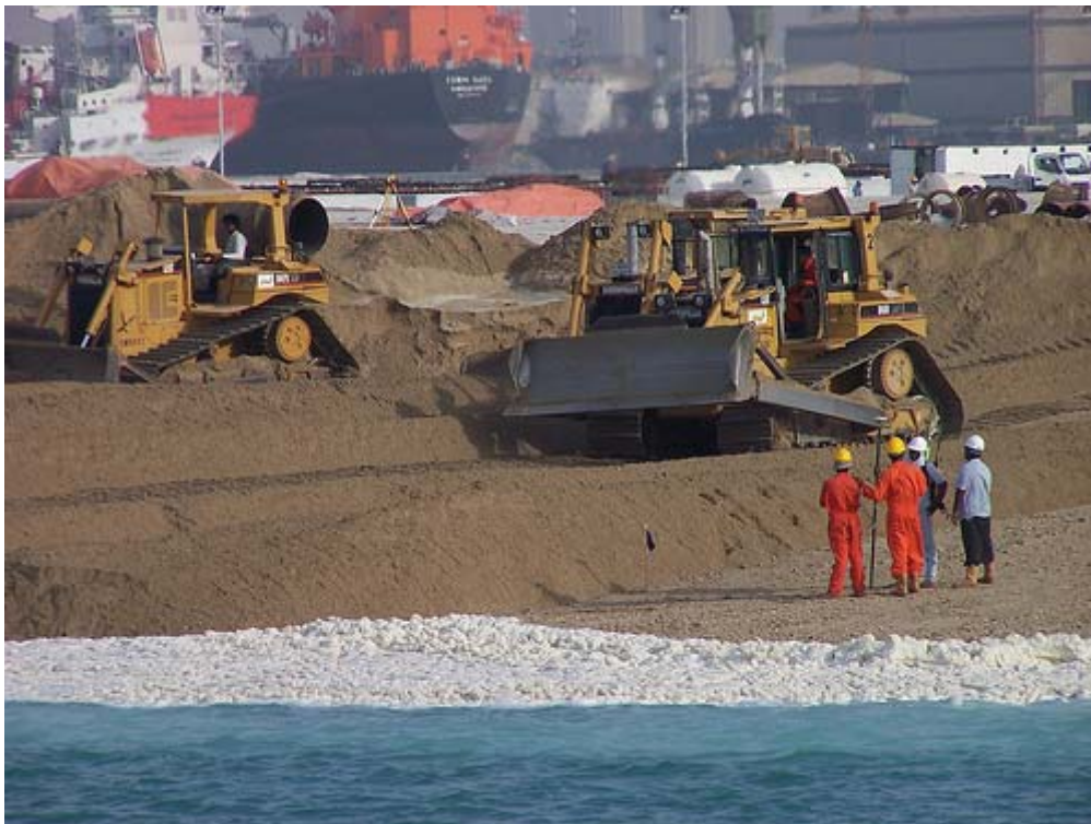
Figure 14 | Bulldozer reshaping the discharged sediments in Dubai
