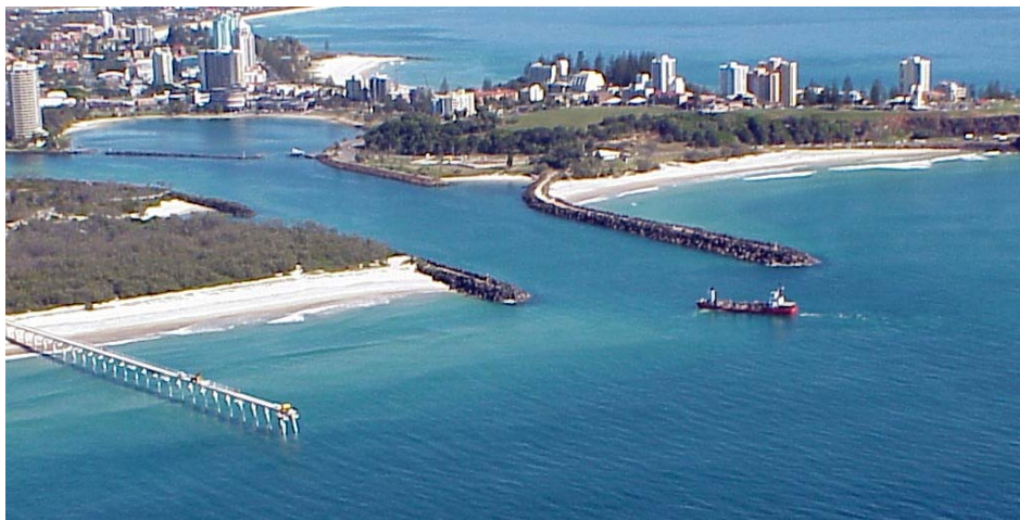
Figure 5 | Interception-mode plant at Tweed River, Australia
