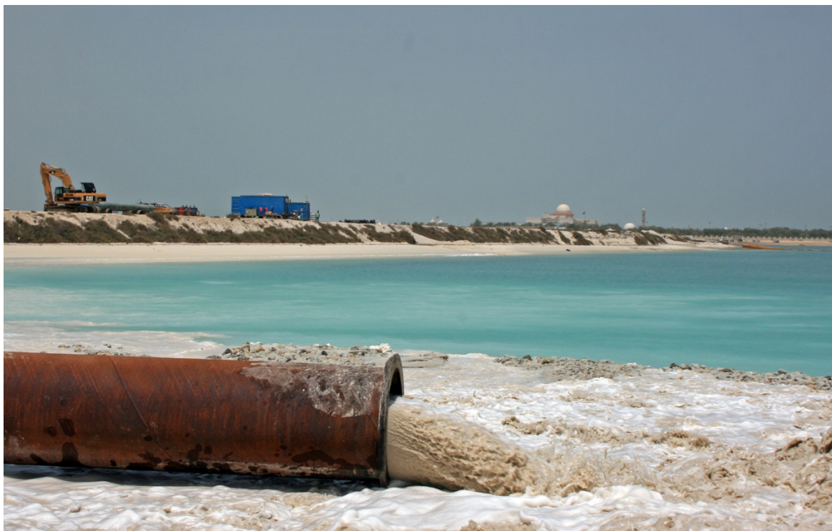
Figure 13 | Sand discharge in a project in Abu Dhabi
